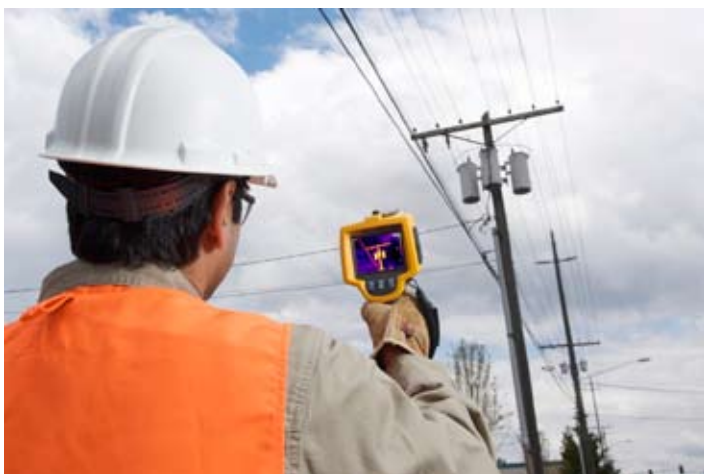
Utility worker scans pole top transformers efficiently and from a safe distance. Printed with permission. Fluke Corporation
