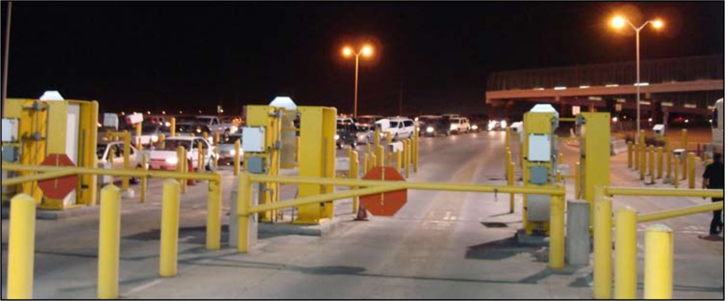
A typical view from Primary Inspection toward oncoming traffic. Good uniformity and a smooth transition zone to darkness beyond are critical to an officer's ability to perceive oncoming threats.
